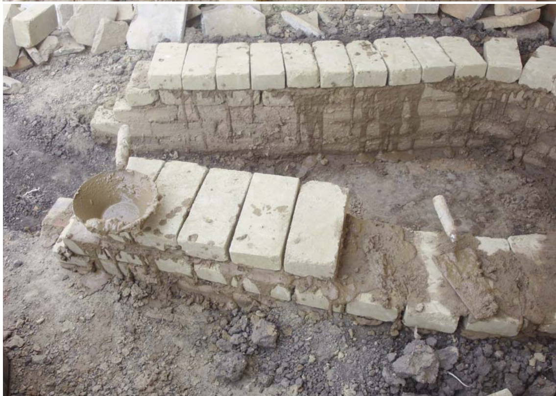
Planşa VII / Plate VII (foto 17-18): Construcţia cuptorului 2 / (photo 17-18): Construction of furnace 2.
